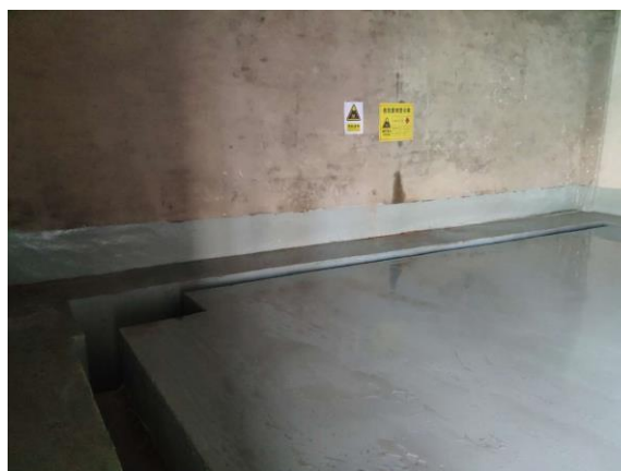
危废暂存间溢流沟
